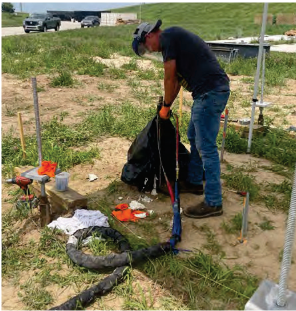
Figure 5.11 Injecting PolyLevel PLSI400H into the soil.
