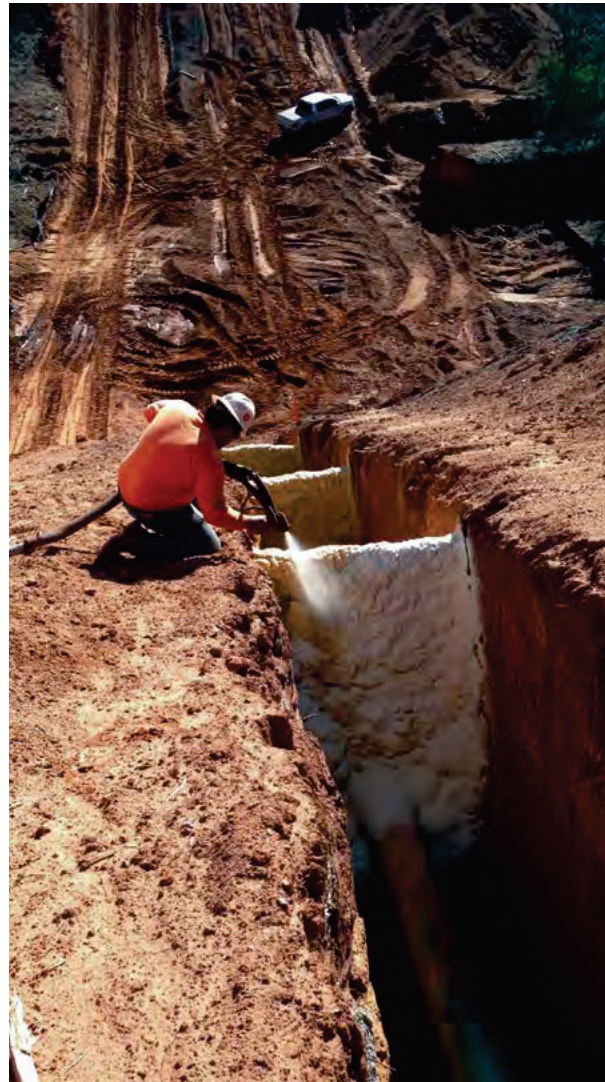
Figure 5.10 Placement of polyurethane foam trench breaks
