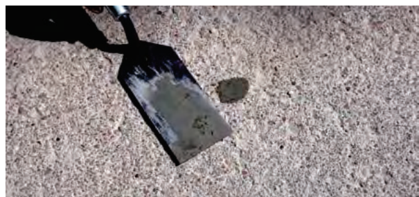
Figure 5.18 Patching the injection hole
