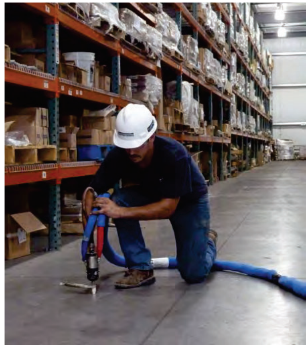
Figure 5.6 PolyLevel stabilizes warehouse floor slab
