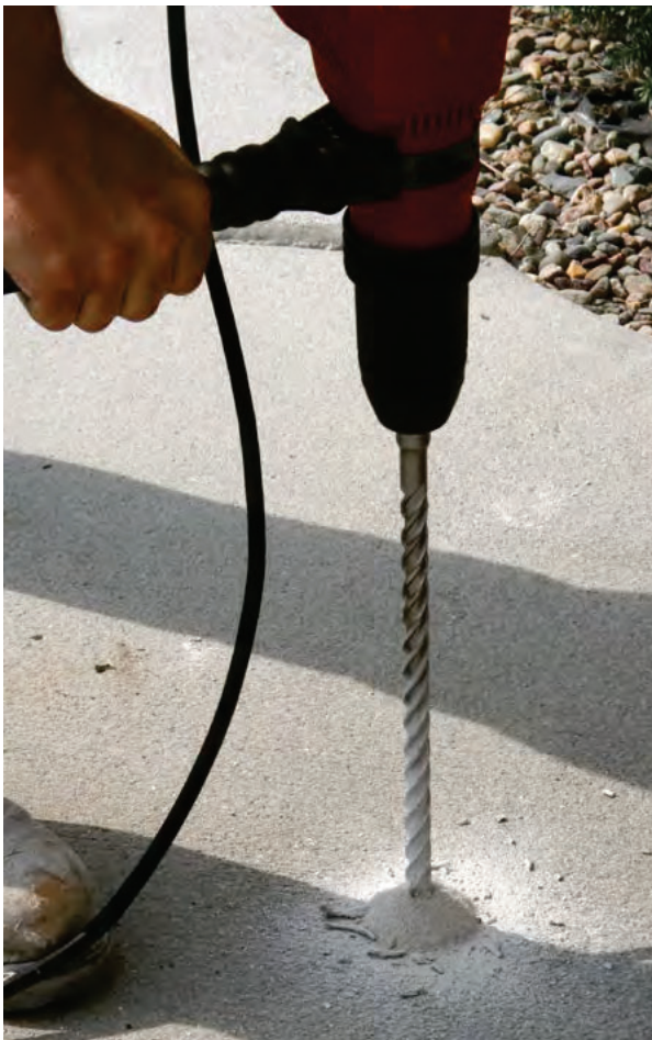
Figure 5.16 Concrete slab drilled to provide access holes
