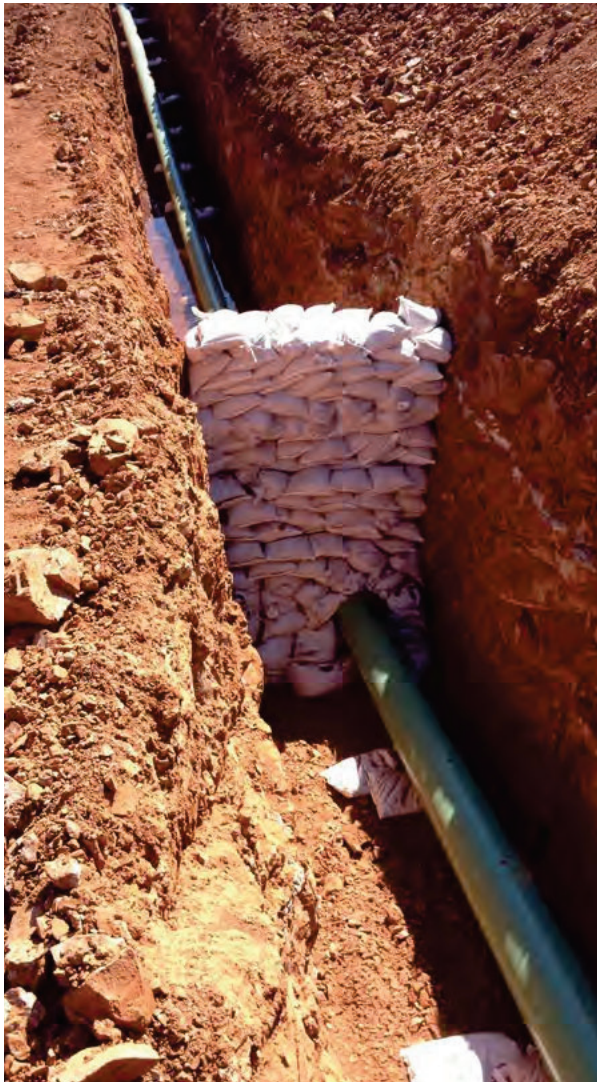
Figure 5.9 Sandbag trench breaker for pipeline
