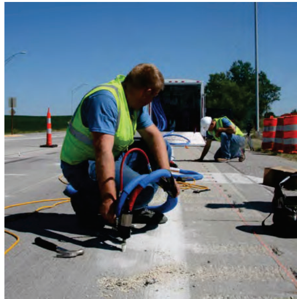
Figure 5.14 Monitoring pavement lift with string lines
